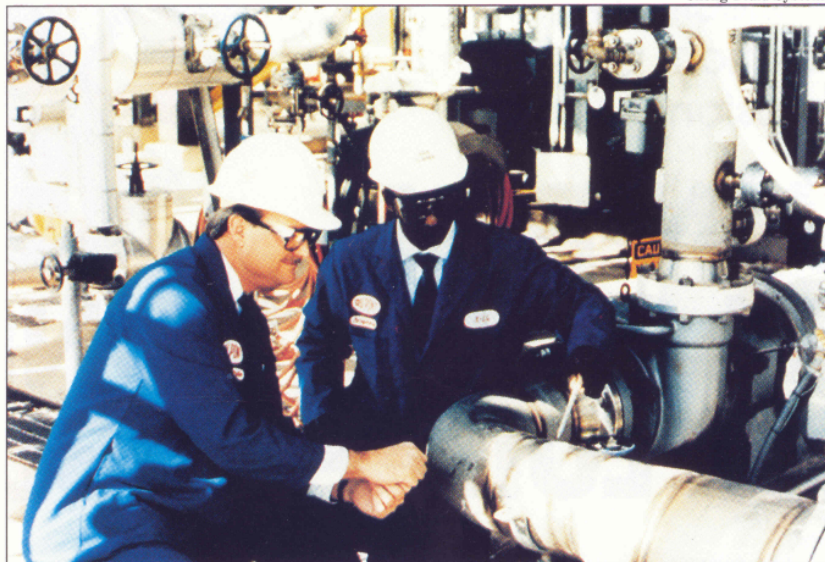
Plant operators at Du Pont's Beaumont facility examine the pipe elbow (bottom of photo) where the CRV is installed, protecting a downstream mag-drive pump
